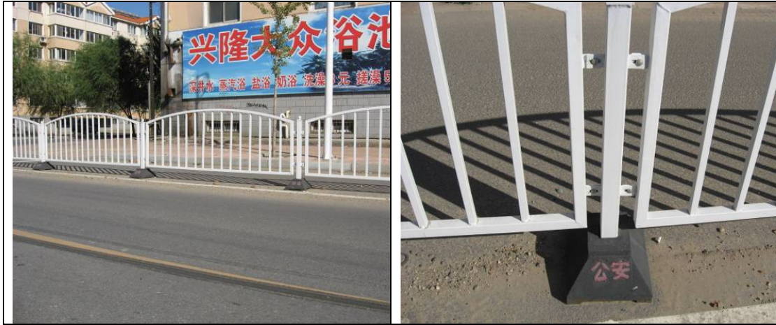
Figure 6-3: Jinzhou Separator with Post and Base Detail
